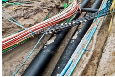
Lay Fiber Optic Cable
