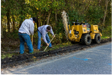
Lay Fiber Optic Cable
